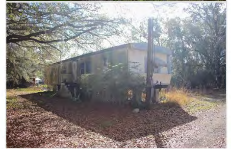
Mobile Home with well & septic (uninhabitable)
